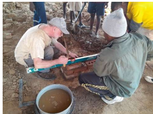
in Zimbabwe with young men learning bricklaying.
